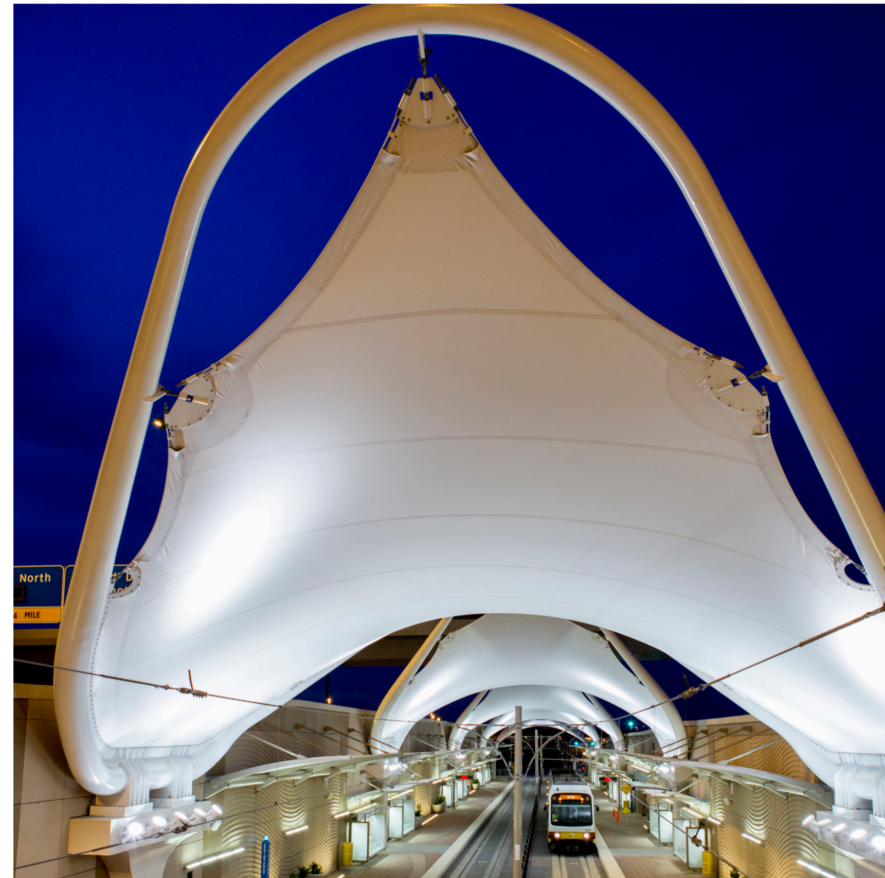
Perspectiva exterior. Dallas Fort Worth. DART station. Fuente: www.googleearth.com
