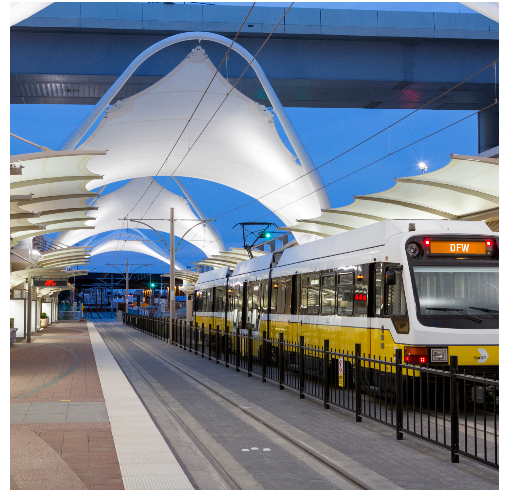
Perspectiva exterior. Dallas Fort Worth. DART station. Fuente: www.googleearth.com
