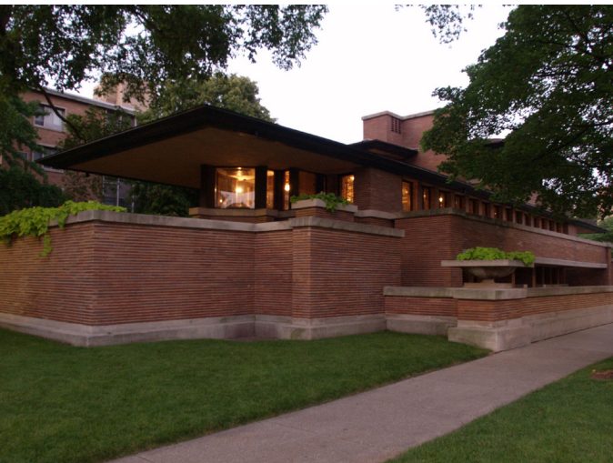
Robie House, Chicago, IL. Frank Lloyd Wright, 1909
