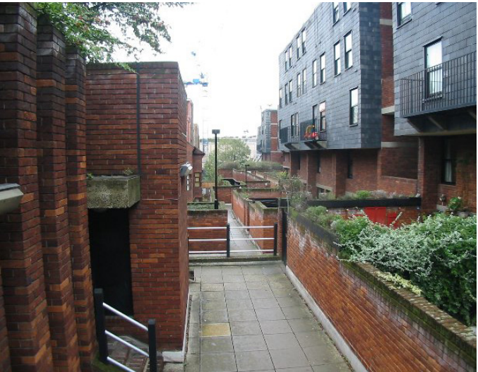
Marquess Road, Islington, UK, Darbourne & Darke, 1971
