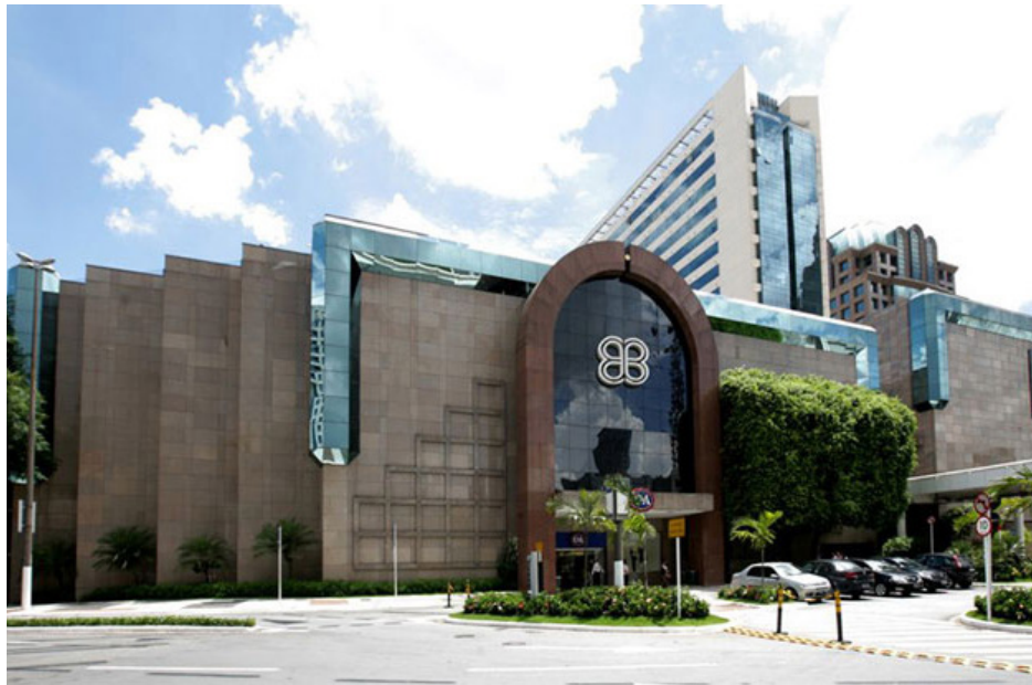
Img. 15. Shopping Morumbi, Arq. Jorge Zalsupin et al, São Paulo, Brazil, fines de 1980s
